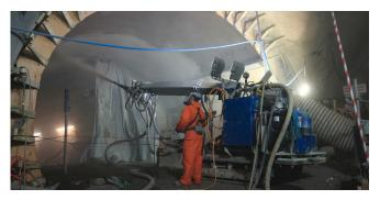
Fig. 1: Shotcrete application in a freshly excavated tunnel using a 5-DoF concrete spraying unit. Image provided by Costain Laing O'Rourke Joint Venture.
